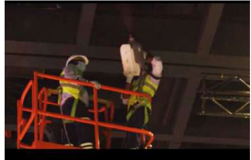
Air change rate in the halls is 8 times per hour. Air extraction in the halls is pre-scheduled and all hall shutter doors will be kept open both before and after the event to assist with air circulation
